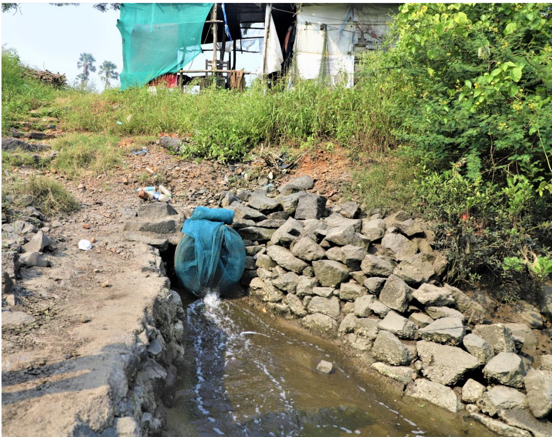
Image 4: Single concrete pipe culvert with fishing net at Panje Wetland.
