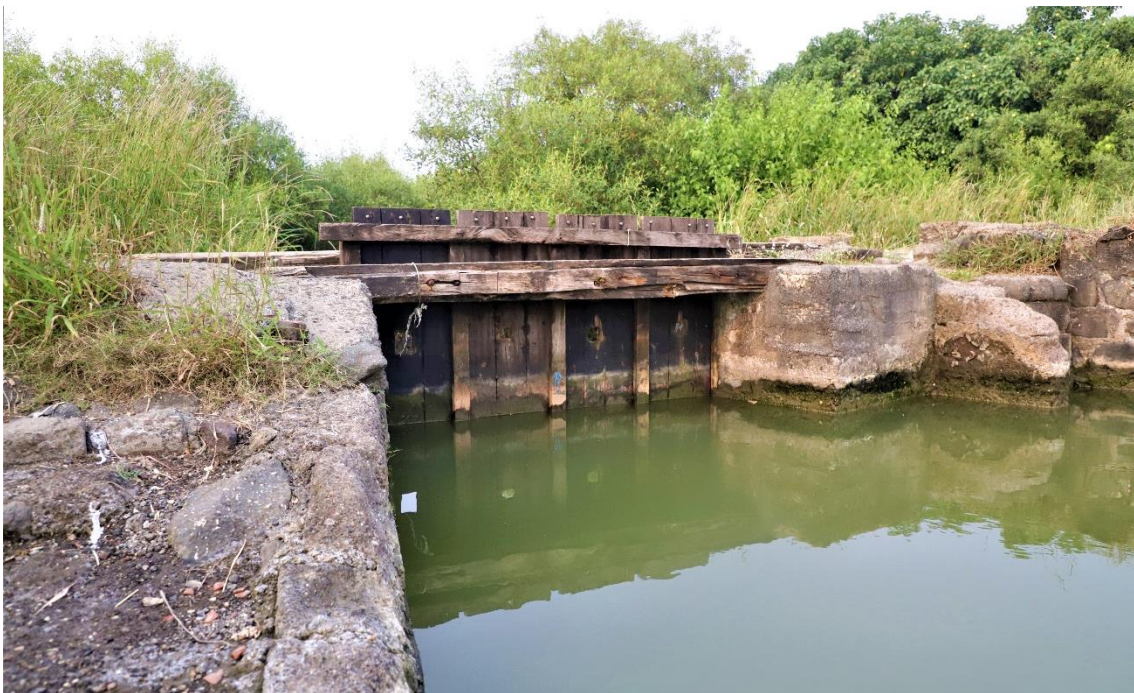
Image 2: Wooden sluice gate on the water channel at TSC.
