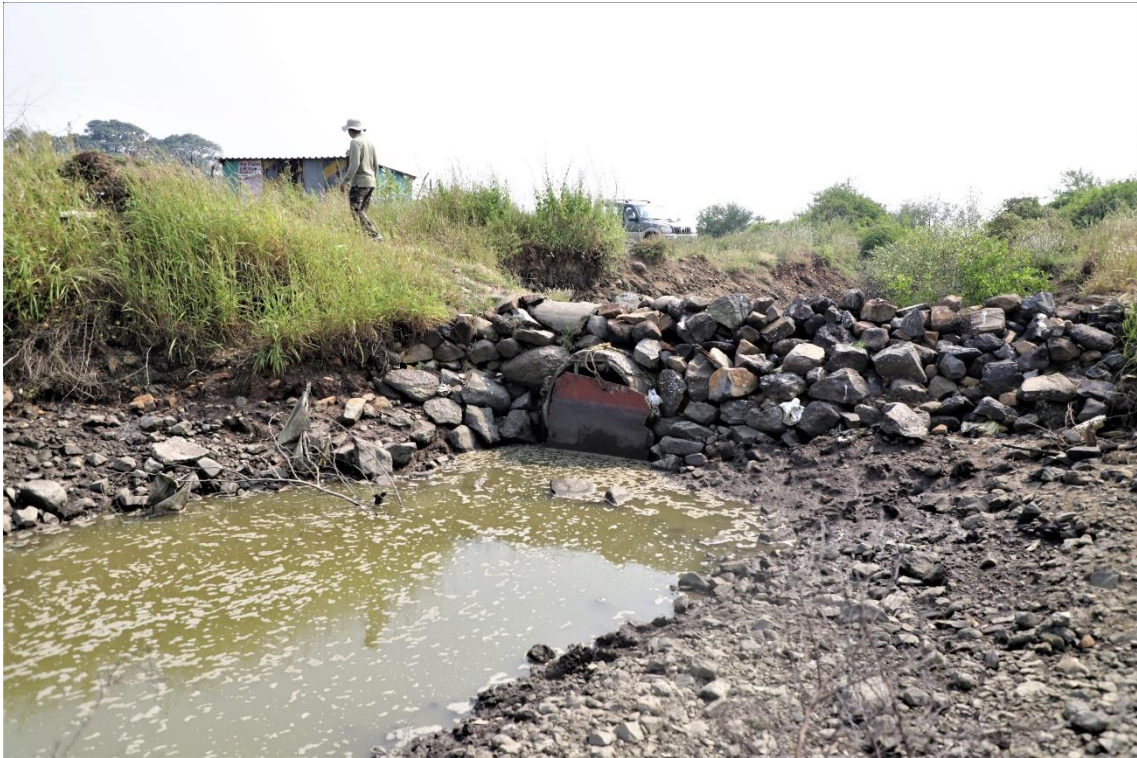
Image 3: Single concrete pipe culvert with a door at Panje Wetland.
