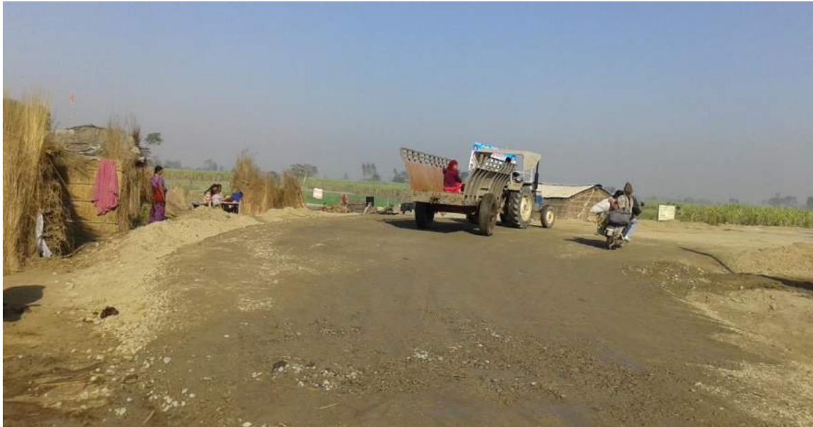
Image 5 Construction of Indo-Nepal border roadway was found under progress everywhere
